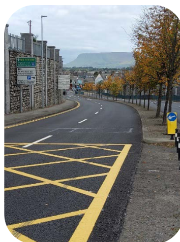
Completed resurfacing works on the N4 looking northbound
