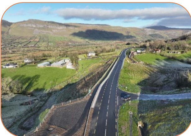
N16 Mainline at Lugatober
